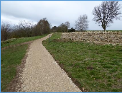
The re-built drystone wall leading up from Hartley Lane alongside a re-surfaced foot path, part of a new 3km accessible route across the top of Leckhampton Hill.
