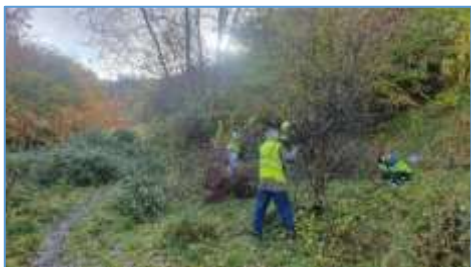
During the work . . .
