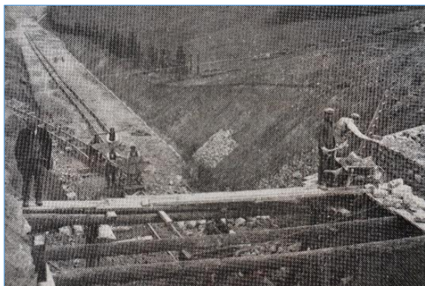
Daisybank bridge under construction (Photograph - the late TF Coke)
