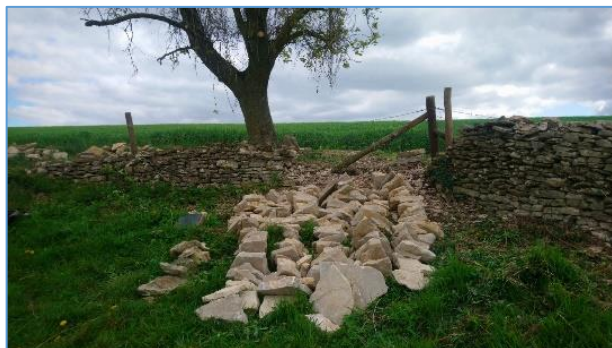
New stone now stacked on the "right" side of the wall
