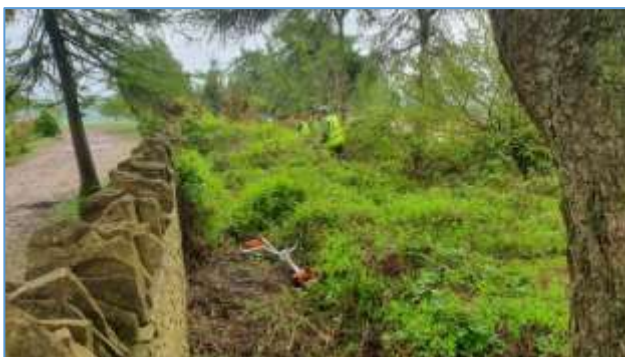
Clearing unwanted growth from the Cotswold Stone Wall
