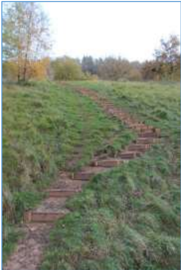
New steps from Bridge Car Park
