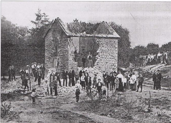
Two stages in the demolition of Tramway Cottage, 15 July 1902. On seeing the mob approach, the quarry foreman and his family fled. The house was ransacked and the building razed to the ground. In 1906 Dale rebuilt the house on the same spot, and on Good Friday 1906 an angry crowd repeated the destruction of fences and cottage. G.B. Wilts read the Riot Act and in due course eight men were tried at Gloucester Assizes.
