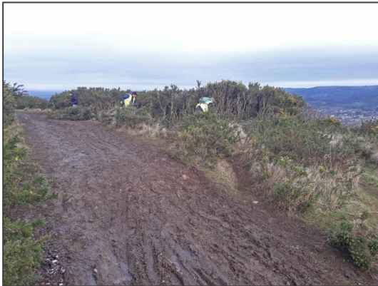
Removing Gorse alongside the Cotswold Way
