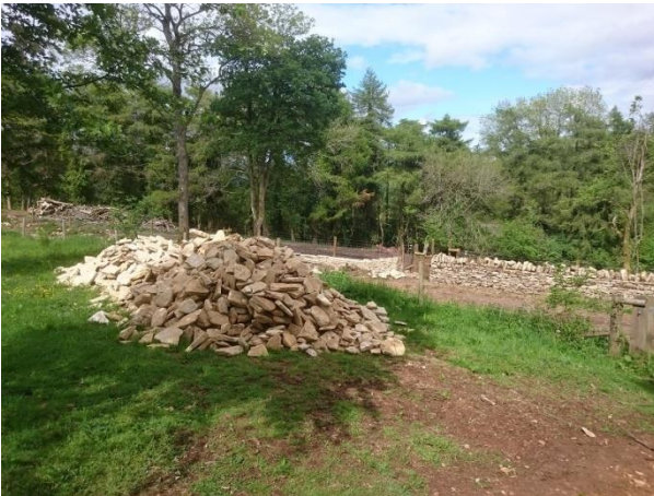
Ready to start building the wall
