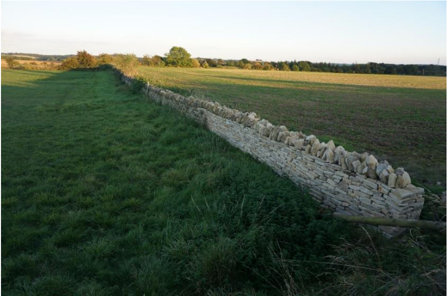
The finished section of wall by the Hill Fort
